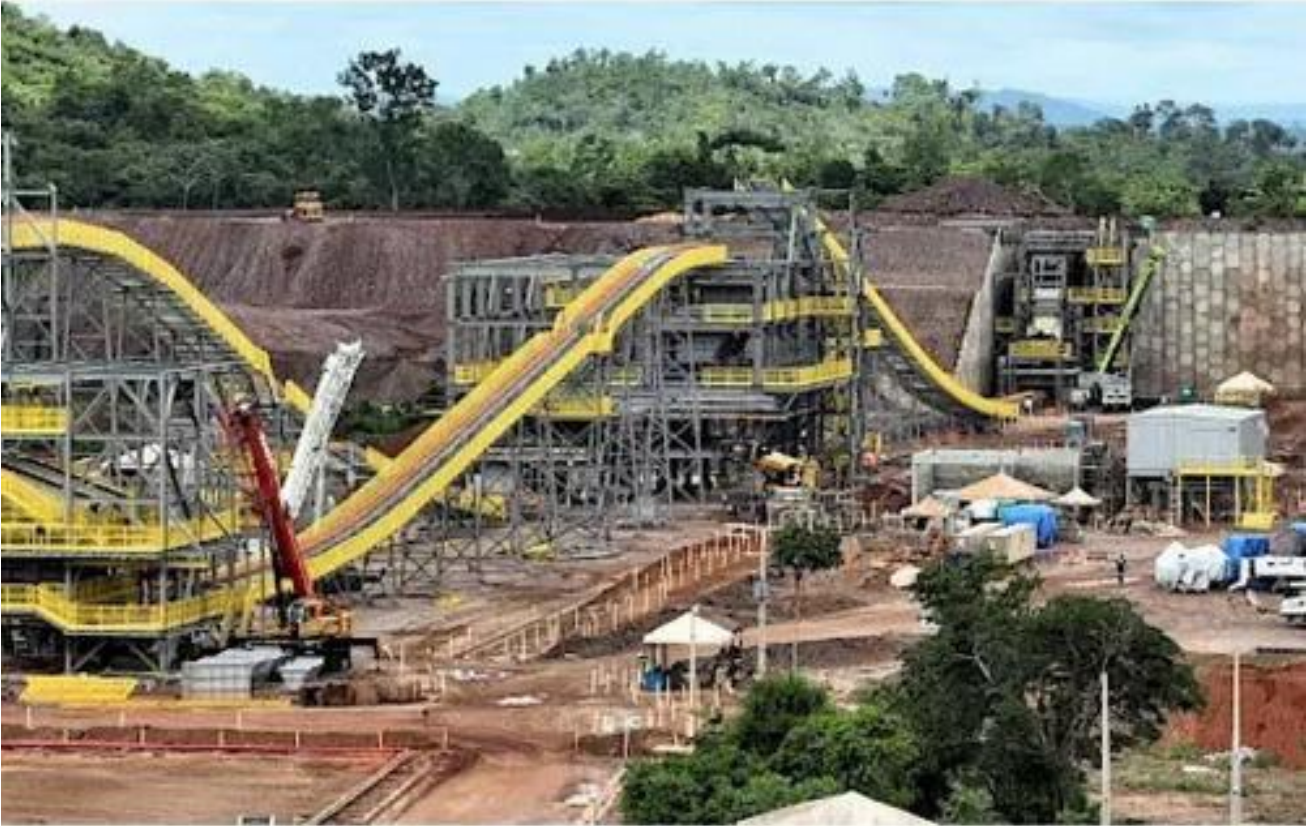
Construction of Ero Copper's Tucumã project
