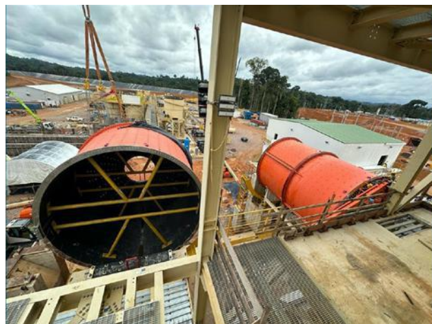
Construction of the Tocantinzinho project, by GMIN
