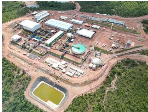
Serra Verde mining industrial plant
