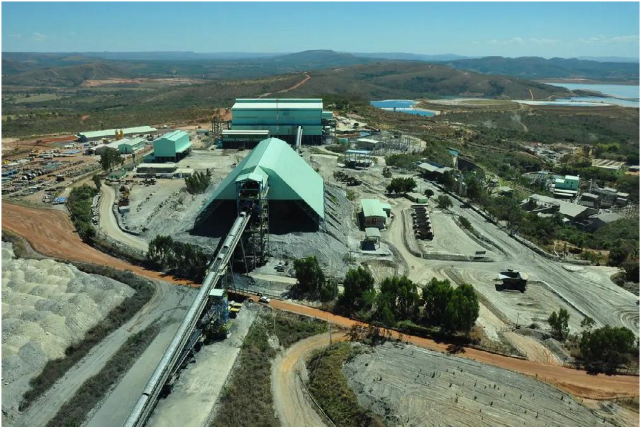
Kinross Morro do Ouro mine facilities in Paracatu
