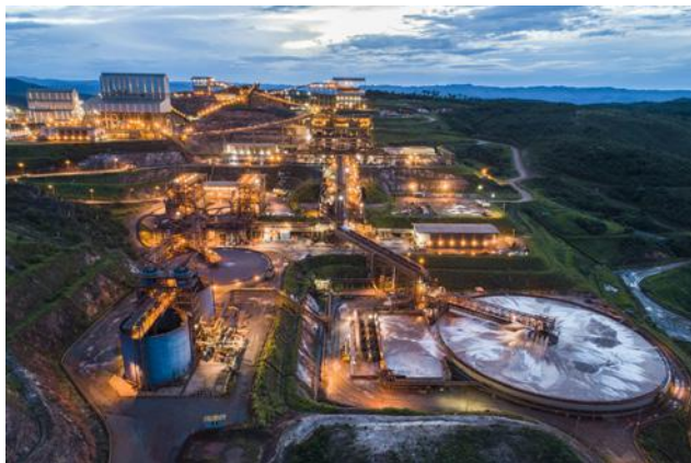
Anglo American's Minas-Rio complex
