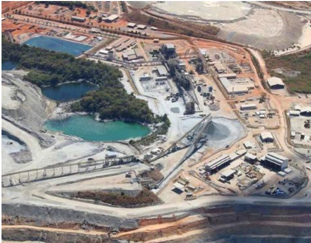
Lundin Mining's Chapada Mine in Goiás
